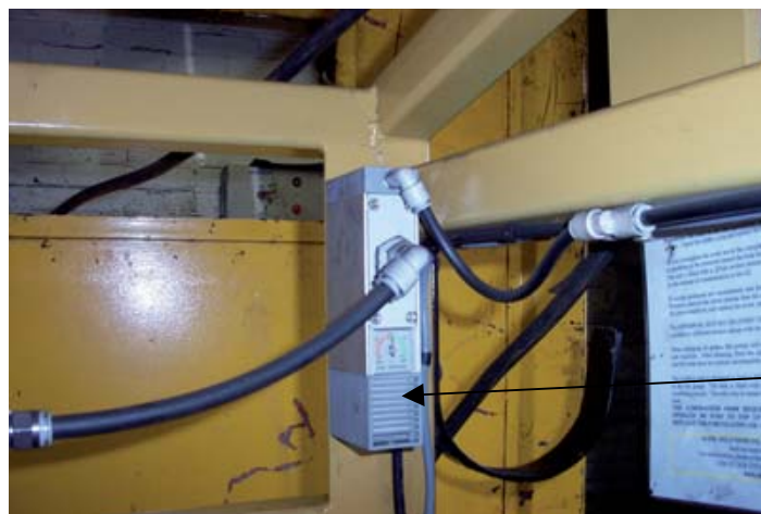
Vacuum generator should not emit vapour
